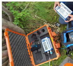
Figure 5.0 A technologist monitoring vibrations near a construction site.
